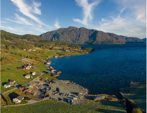
CONSTRUCTION STATUS PER OCTOBER 2023
