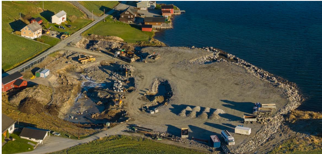
Ongoing constructions at Tingvoll
